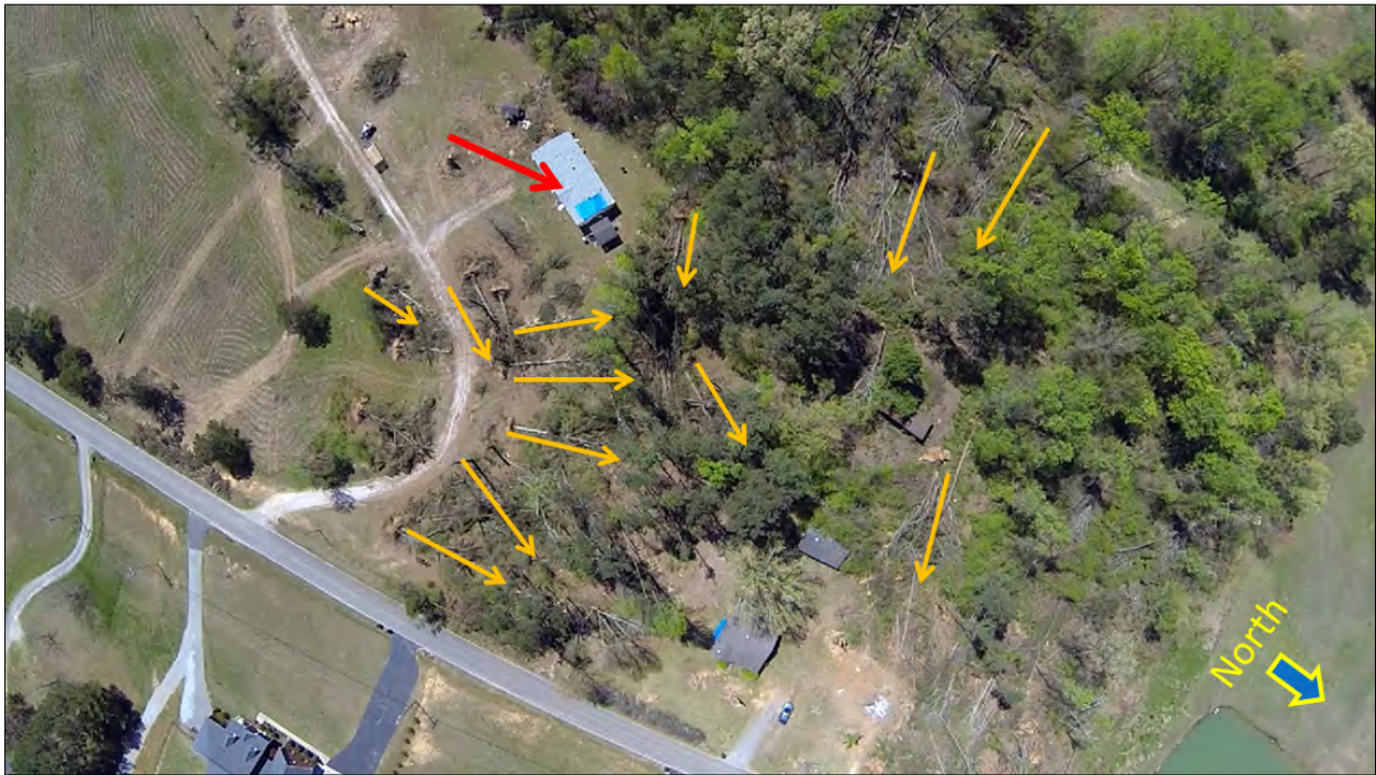
Figure 12: Damage near the middle of the Pricville tornado track on 5 April 2016 from Flight 2. Orange arrows indicate direction trees fell; red arrow indicates roof damage. North arrow indicated in bottom right.
