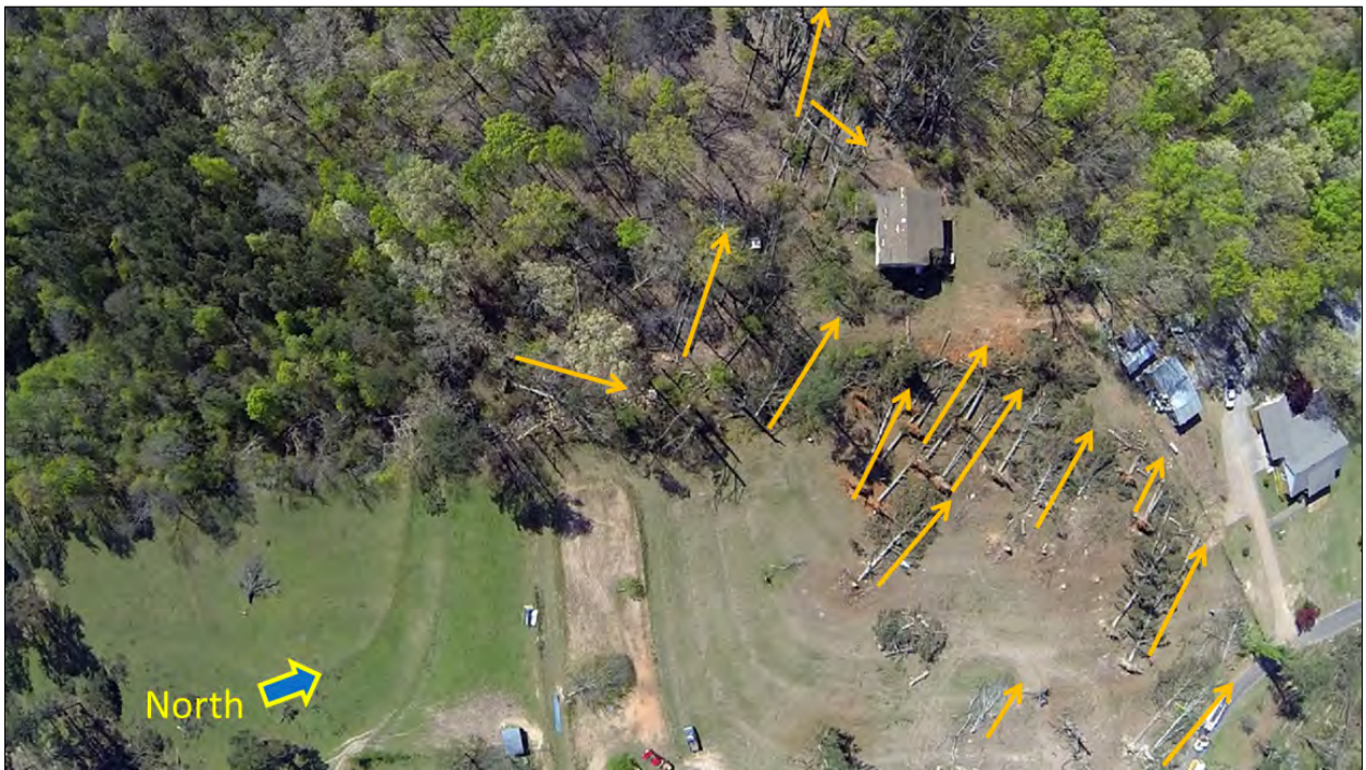
Figure 14: Damage near the middle of the Priceville tornado track on 5 April 2016 from Flight 4. Orange arrows indicate direction trees fell. North arrow indicated in bottom right.
